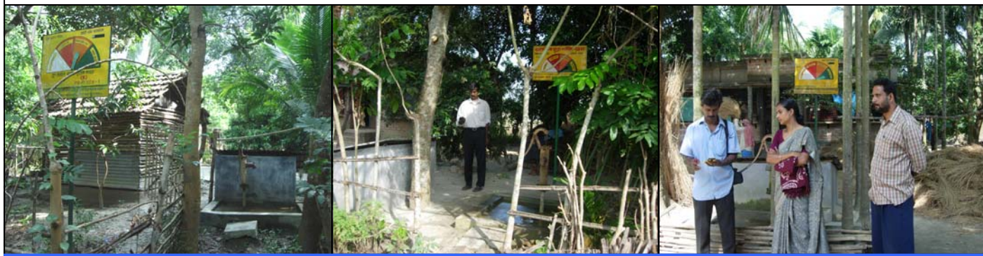
Left: PW46KDK1-R was built to replace PW01KDK1. Center: PW47KDK7-R replaced PW08KDK7. Right: PW48KLS7-R replaced PW18KLS7.
