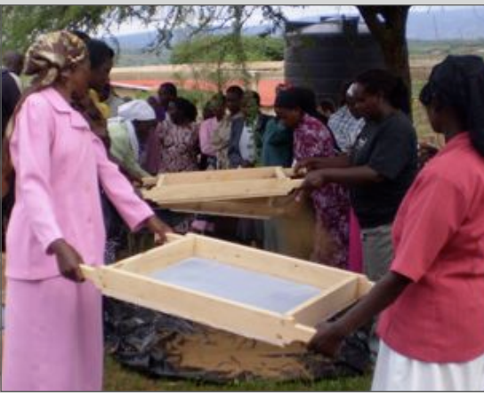
Local sand and gravel for filler material.
