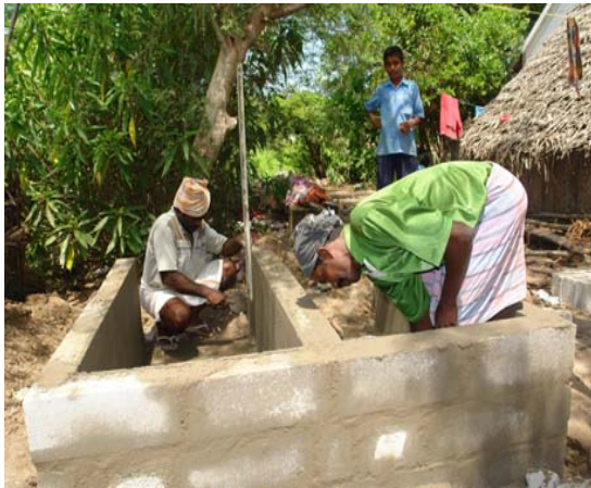
The chambers under construction
