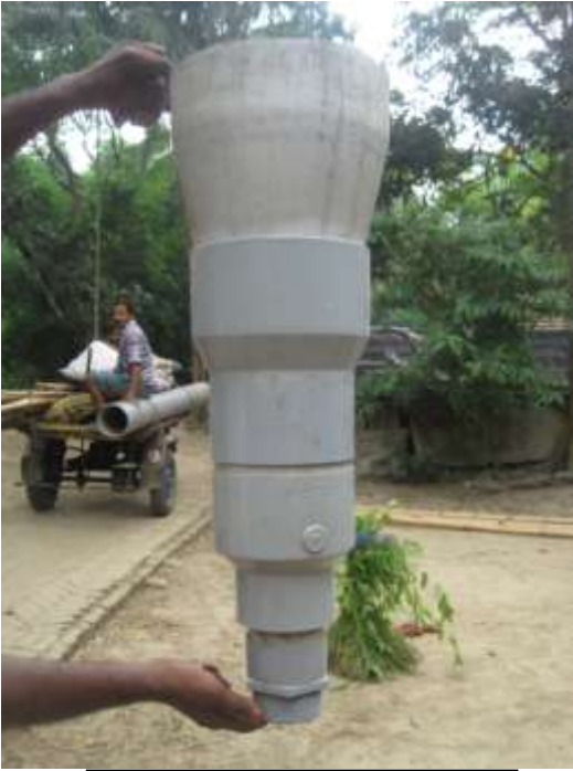
This reducer is fixed on either end of the 10foot pipe.
