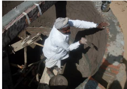
Ongoing construction of Taanka at Madhogarh village, Diyatra
