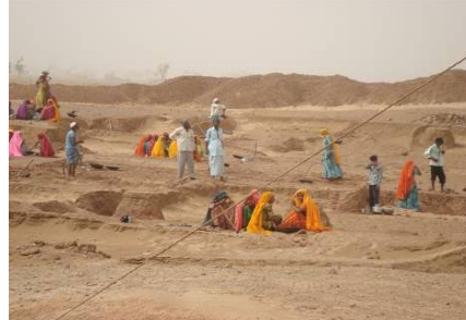
Desilting Work in Progress in Kesarpura Naadi (village pond)
