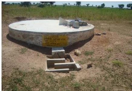
Taanka constructed with rainwater harvesting technique
